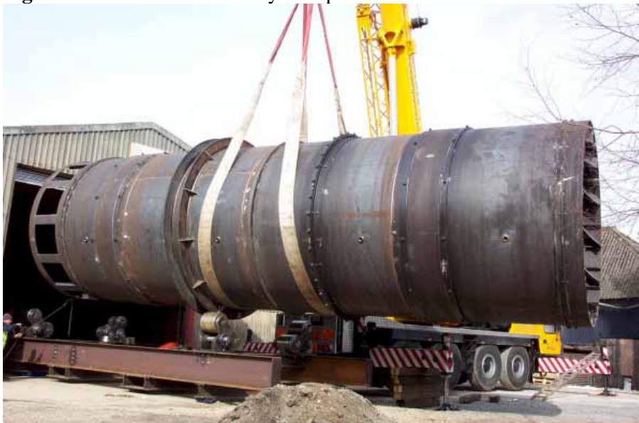
Figure 1. Installation of Rotary Composter
