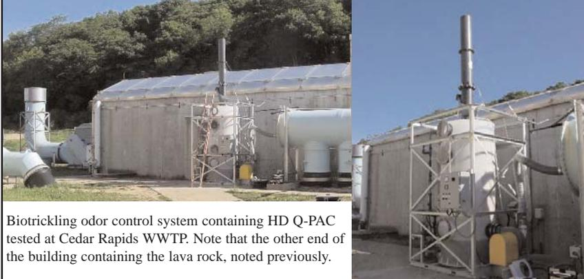
Biotrickling odor control system containing HD Q-PAC tested at Cedar Rapids WWTP. Note that the other end of the building containing the lava rock, noted previously.
