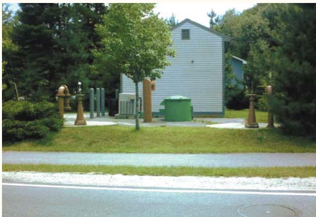
Windy Point Pump Station with nearby house in background
