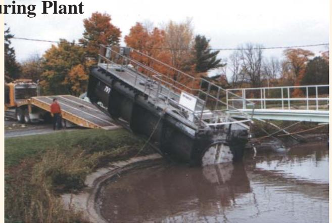
The three million gallon lagoon has two five horse-power splashers operating during the Department of Environmental Conservation (DEC) Summer Permit discharge conditions from May to November. During the summer, the undiluted whey-waste water in the lagoon is drawn down and sprayed onto the adjacent meadow, which is owned by the cheese manufacturer.
