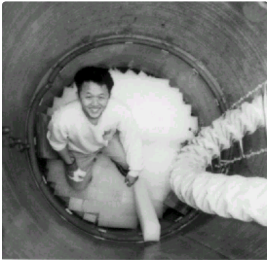
Figure 6. The author installing HD Q-PAC ®
