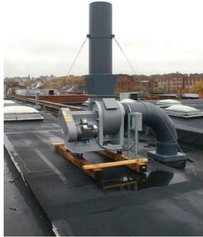
Figure 2 – Roof Mounted Exhaust Blower
