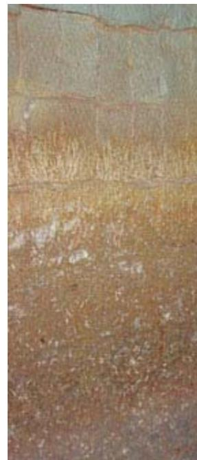
**Figure 4. Distinct settlement lines and impressions into insulation along inside of the canister walls caused by collapse of the saddle**
