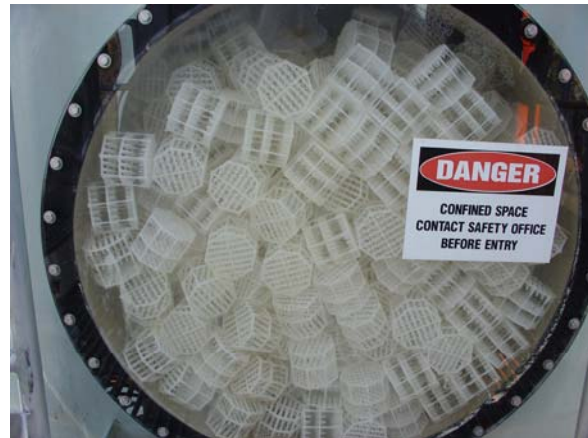
Q-PAC ® Random Dumped Into Odor Control Scrubber
