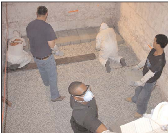
Installation of MLM® on 25-mm ceramic ball support
